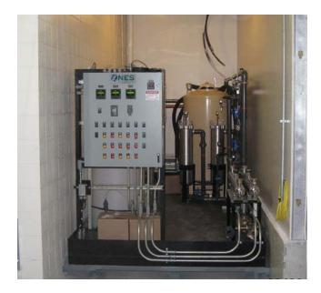
Project Objectives: Treat Groundwater for Multiple Contaminants using UV, Chem-Ox, and Carbon Adsorbtion Technologies in a footprint limited to the size of a parking space.
